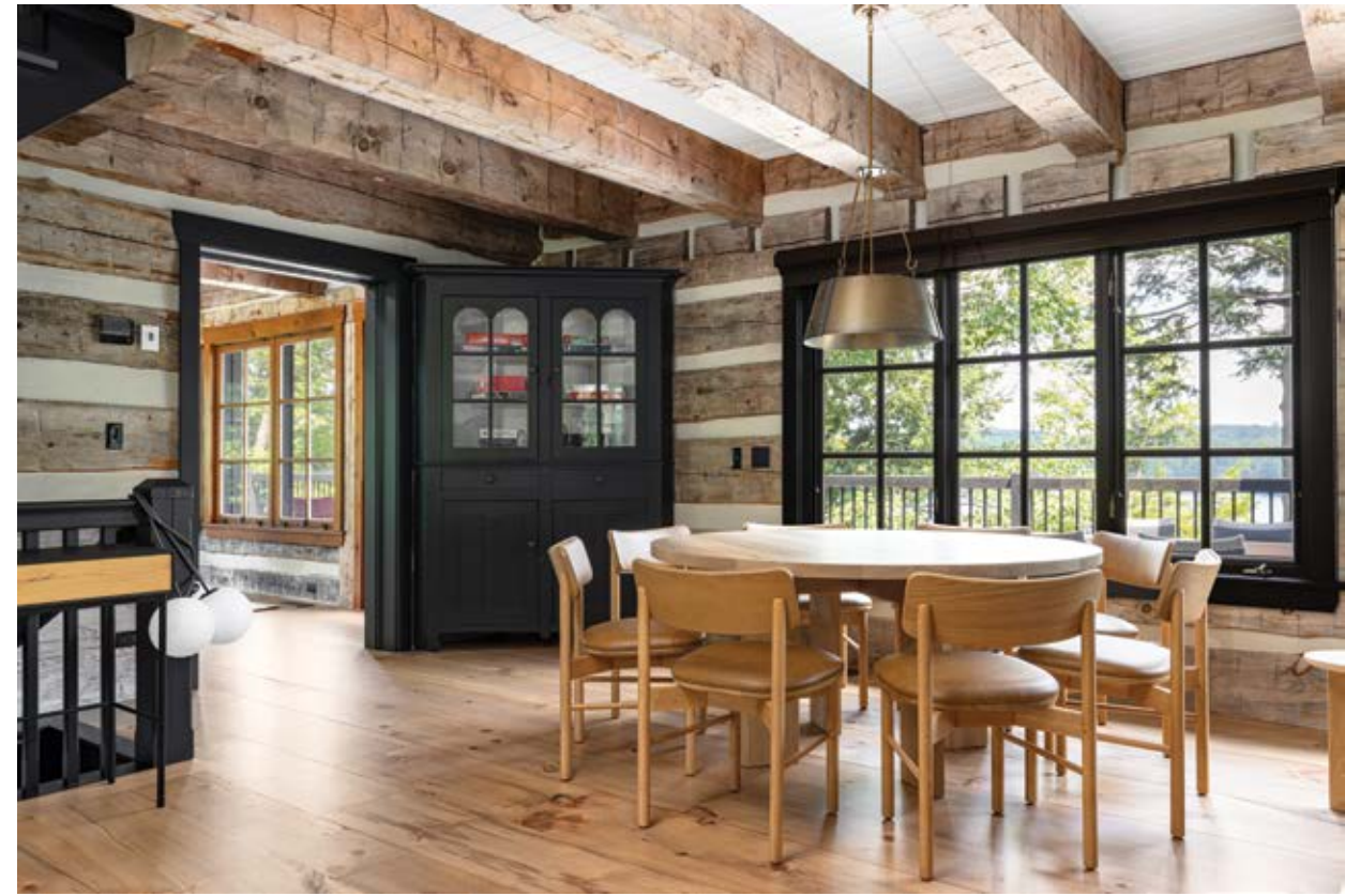
ABOVE: Natural Prestige Log Homes Ltd. supplied the large timbers, hewn from newer pine logs, to support the second floor, as required by new construction regulations. RIGHT: Visible above the windows are old floor joist notches from one of the century-old cabins dismantled to create this home. OPPOSITE BOTTOM: Stone fireplaces in the kitchen and living room were built to mirror the style of masonry in late 19 th century cabins.
